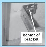
FIG. 4-2 Mounting brackets.
